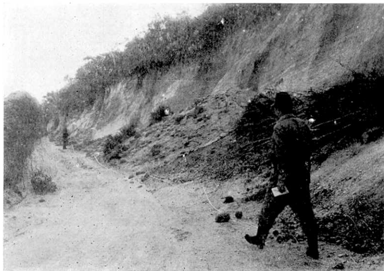
Fig. 14. Landslide at Kozu-sima.
