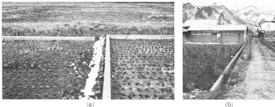
Fig. 43. a: Cracks in concrete levees between rice-field, looking eastward. Note that there are three open cracks in the levees in a N-S direction whereas the E-W levee is free from cracks. Photograph taken Feb. 21, 1967.
