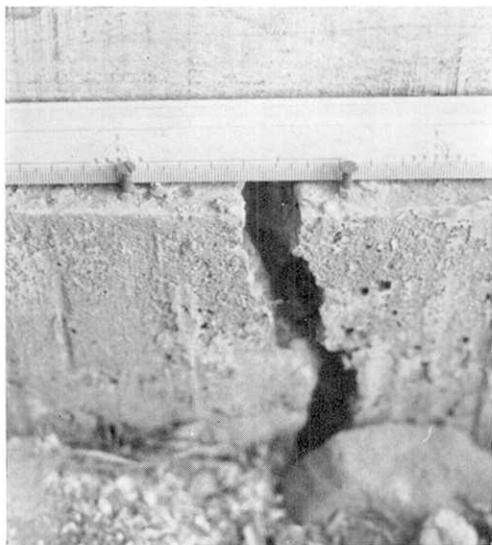
Fig. 19. Method of type Ic-s at Station F<sub>2</sub>-b (In), where a crack occurred crossing a concrete base of a wooden house. Photograph taken Jan. 26, 1967.
