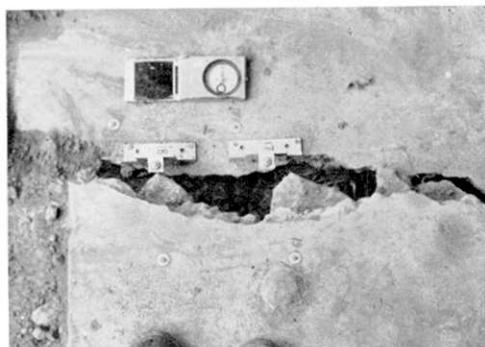
Fig. 13. Broken concrete slab at locality F<sub>1</sub>-a, showing left-lateral displacement of crack A on Sept. 16, 1966. The same crack in April, May and June, 1966 was shown in Fig. 6 in the first paper. Oblique view is given in Fig. 27. Width of clino-compass is 6.5 cm.
