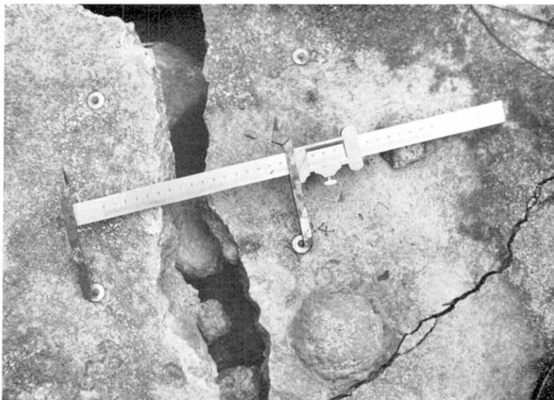
Fig. 18. Method of type Ic-w at Station F<sub>1</sub>-a, D. The concrete slab on the left (north) tilted northwards by subsidence of northern side.
