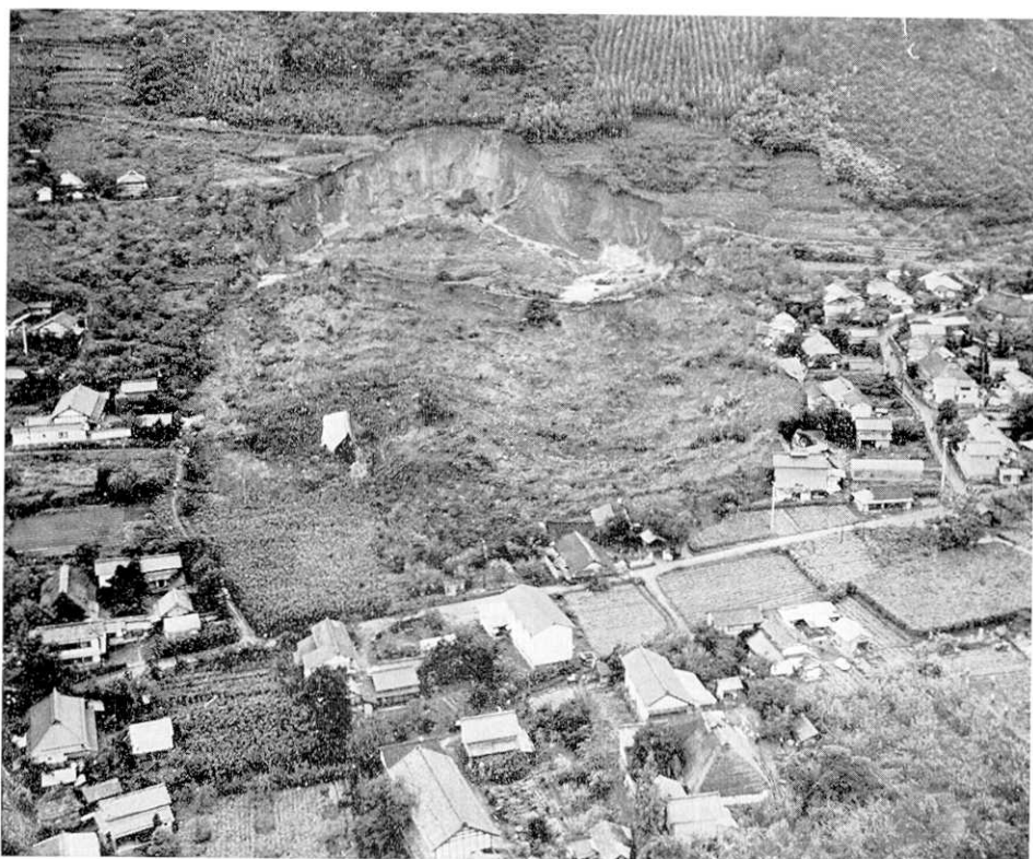
Fig. 6. An aerial view of the landslide at Makiuchi, an hour after its occurrence. Underground water pouring out from the curved scar at the head of the collapsed area is dammed up behind the ridge of the rotated mass. Mulberry trees intermingled with slid earth draw the flowage patterns to wards the front, similar to a big surface pattern of ropy lava flow. Smaller embayed portion at the top of the cliff collapsed secondly, about 30 minutes after the sliding down of main mass. Photo. by Mr. Sakurai, Shinano Mainichi Press, around 15h, 17th September 1966.
