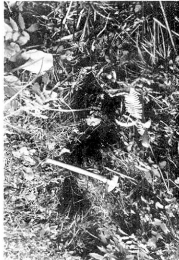
c: Fissure along the foot line of the scarplet
