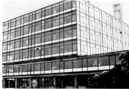
Fig. 6. Outside view of Shimizu City Hall after repairing the broken glass.
