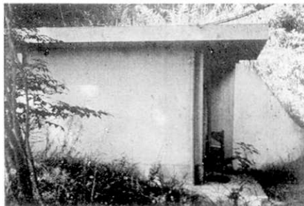
Fig. 3. External appearance of the vault. The seismograph and galvanometer rooms are covered by soil.
