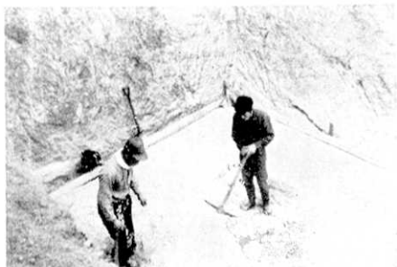
Fig. 1. Basement of the seismograph vault.
