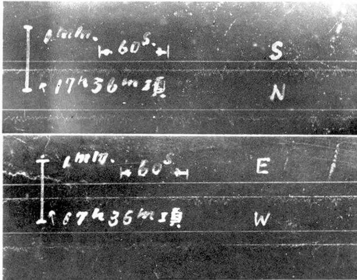
Fig. 17a. Vibration records of the house due to N-E wind.
