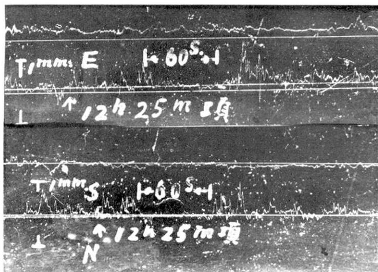
Fig. 18a. Vibration records of the house due to S-W wind.
