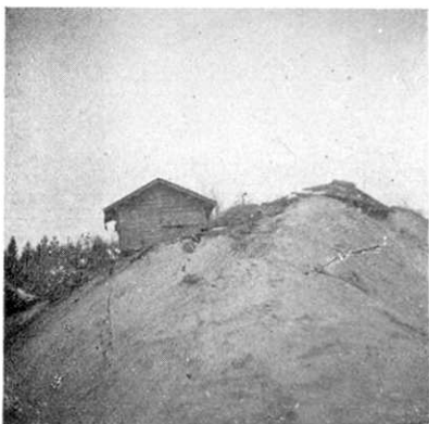
Fig. 7. Slipping of the soil along the weathered layer at the surface of the porphyritic granite, near Kusagyū.
