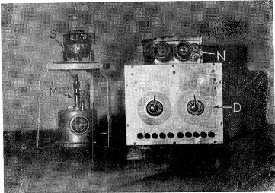
Photo. 1. Remote controlling device for water-tube tiltmeter.
