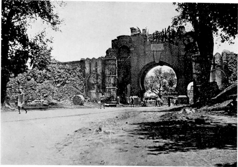
Fig. 19. Gate of Fort Monghyr damaged by the earthquake. N. Nasu, Photo.
