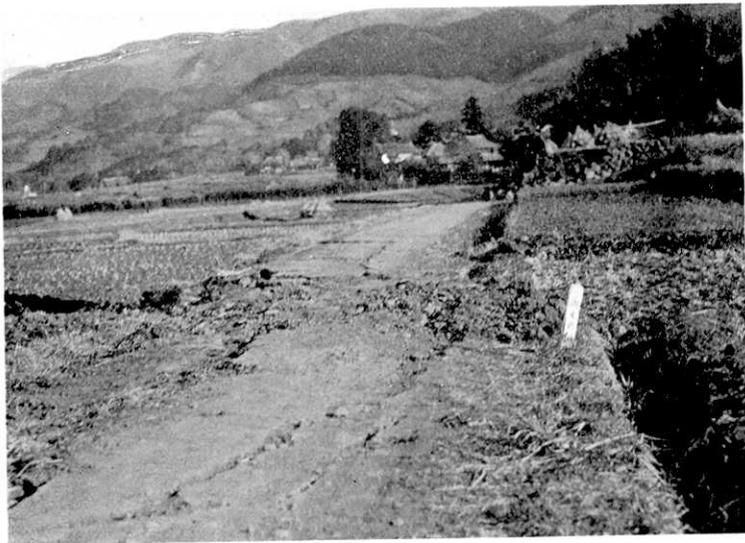
Fig. 32. The horizontal displacement of a small road joining Tanna Nisikata and Takizawa. (H. Tsuya.)
