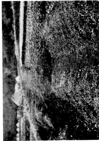
Fig 38. Displacement of a small road in Ukihasi basin, Ukihasi central earthquake fault.
