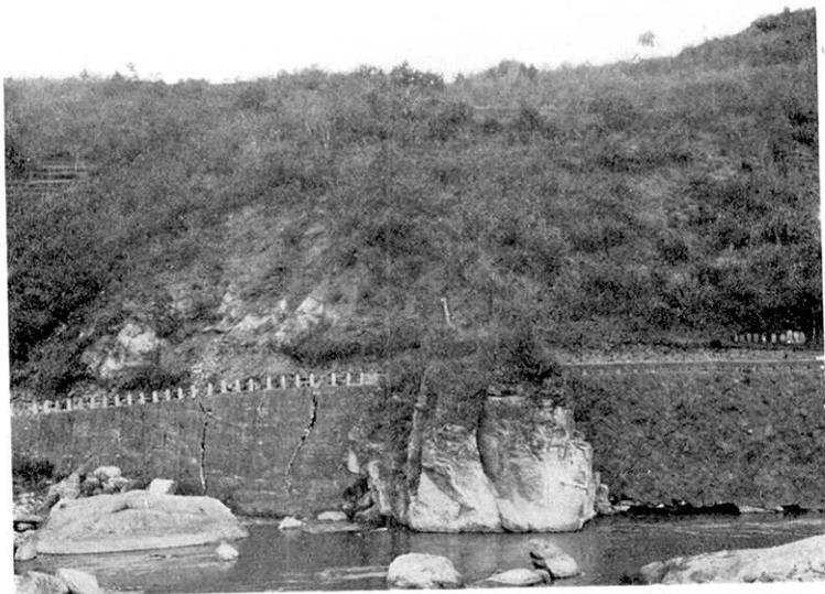
Fig. 44. Earthquake fault cutting through the Ito-Syuzenzi high way, along the Oomi river.
