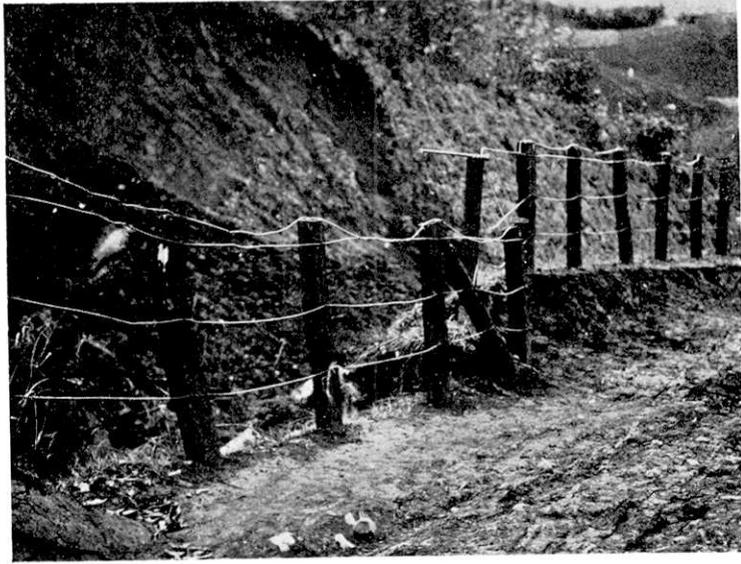
Fig. 31. Displaced fence of Tanna reservoir. (H. Tsuya.)
