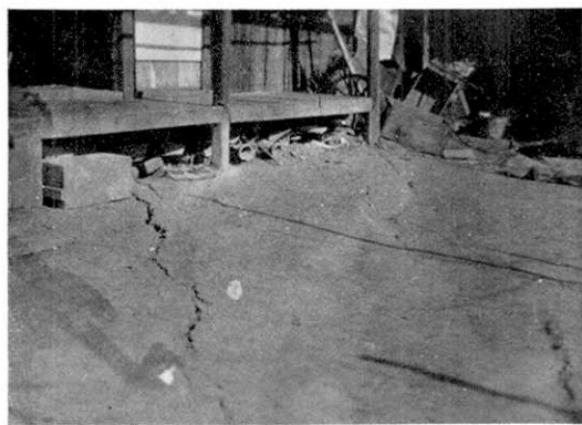
Fig. 7. Crack in the sliding area. (Photo. on the 3rd of February).
