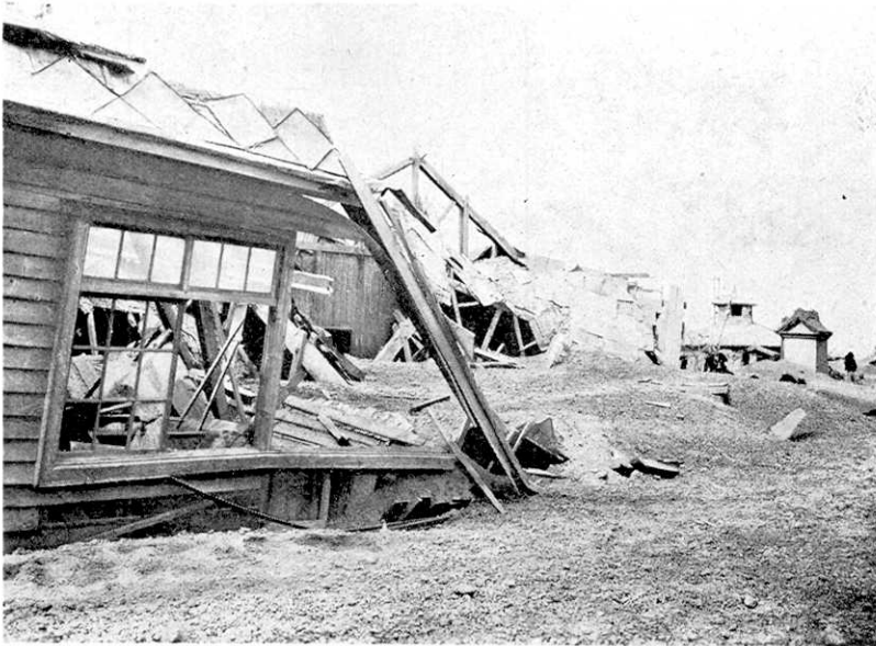
Fig. 2. Houses in Sikabe damaged by the ejecta.
