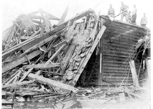
Fig. 13 Broken at the second story.
