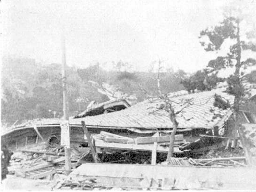
Fig. 29 One storied house roofed with heavy tiles.
