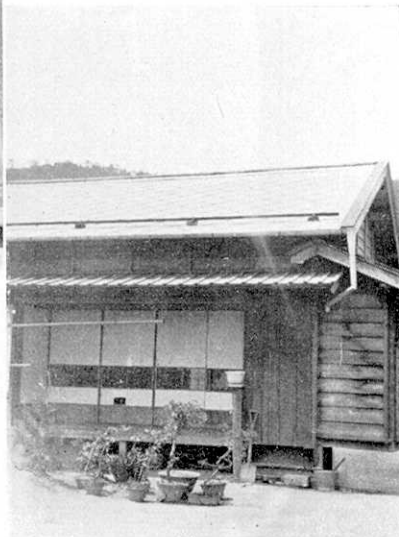
Fig. 32 One storied house roofed with asbestos slates.
