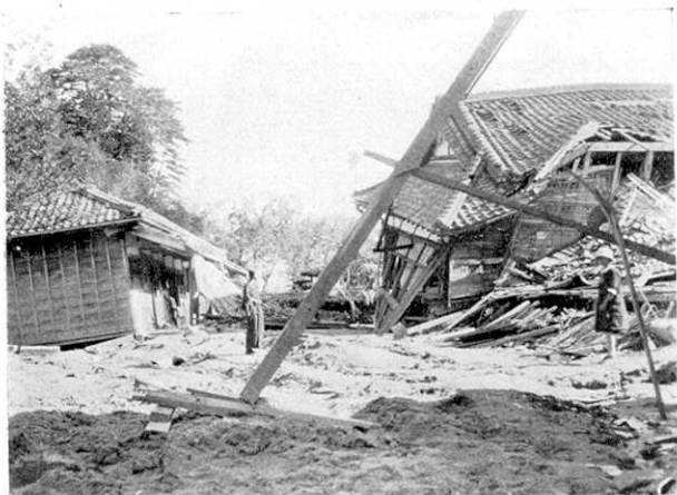
Fig. 19 The Mineyama local court destroyed due to a large fissure on the ground under the building.
