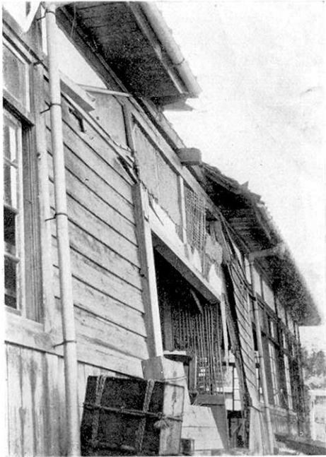
Fig. 23 The porch of the Naka district office.
