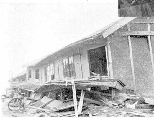
Fig. 31 Two storied house thatched with shingles.
