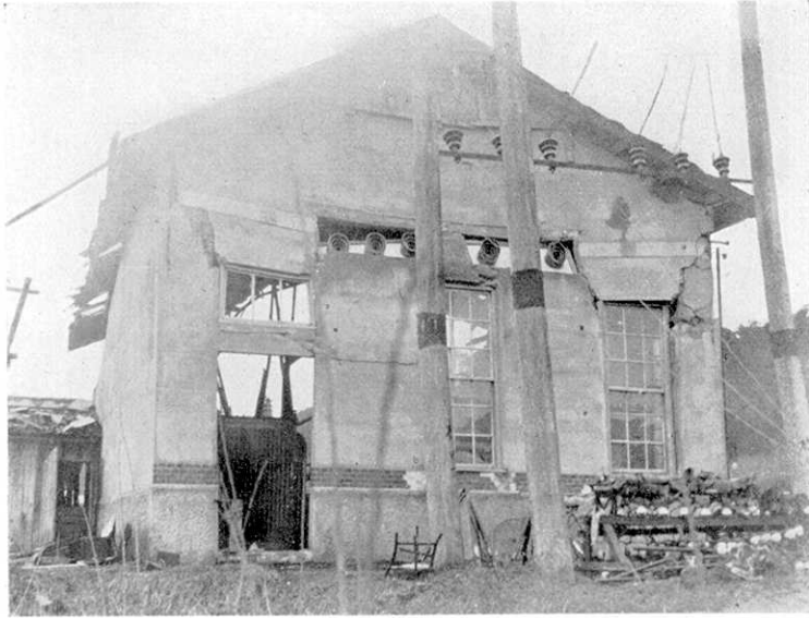
Fig. 27 The Yamada electric substation, constructed of inferior concrete.
