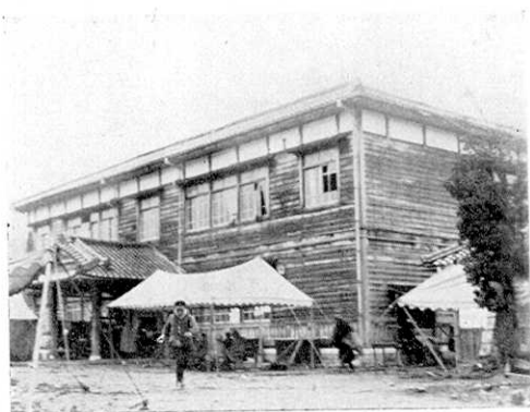
Fig. 24 The Takeda district office remained intact on a soft ground probably for the reason that it is built on a spread foundation.
