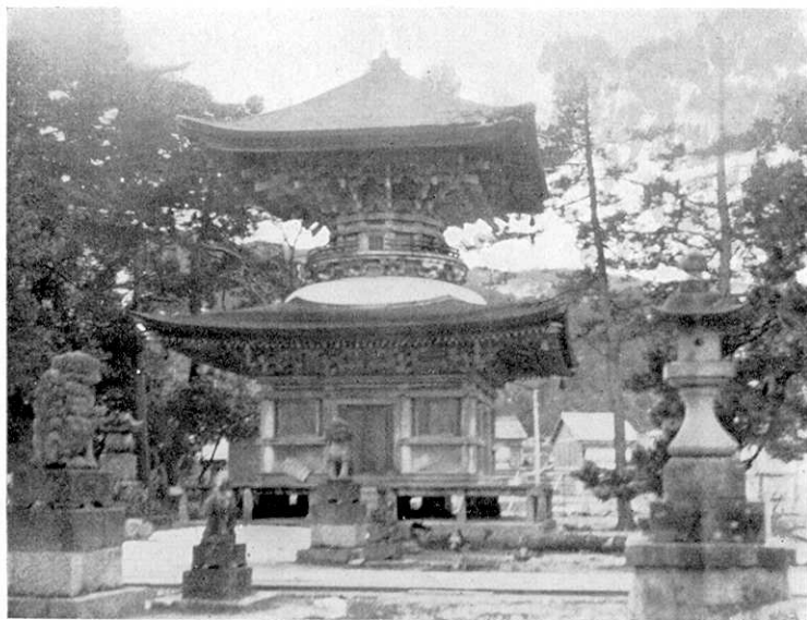
Fig. 25 The "Tahoto" tower of an old temple near Amanohashidate. The central post "Kurin" at the top of the tower fell down.
