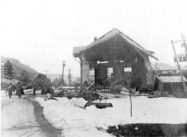
Fig. 28 Another side of the building shown in Fig 27.
