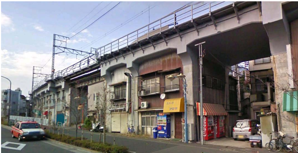
Figure 143 - Oimachi viaduct with large openings for pedestrian crossing
