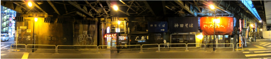
Figure 202 - elevation of one of the triangular lots crossing from east to west
