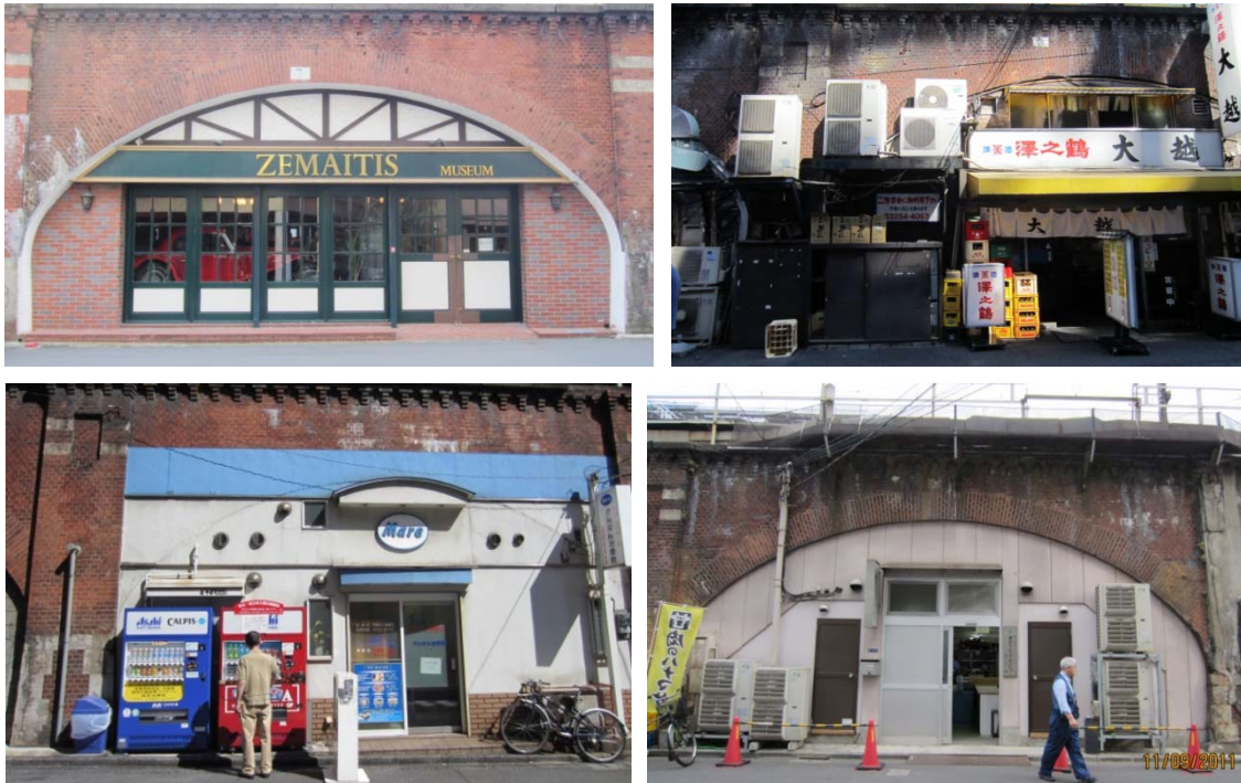
Figure 198 – Kanda's viaduct's spaces along the north section of the brick arches
