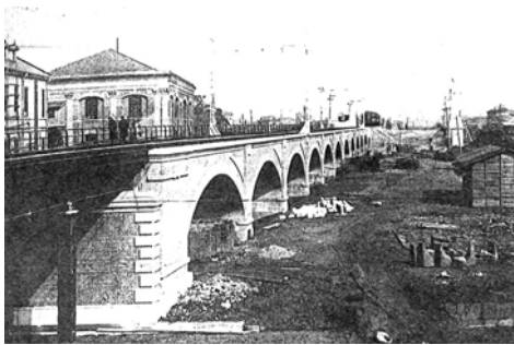
Figure 184 - Sotobori Bashi Bridge looking from Ootemachi Bashi Bridge
