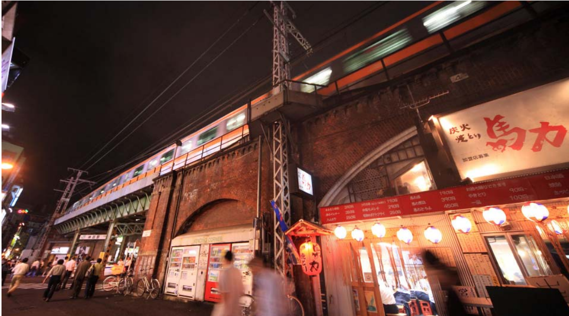
Figure 203 - evening time west side of Kanad's viaduct
