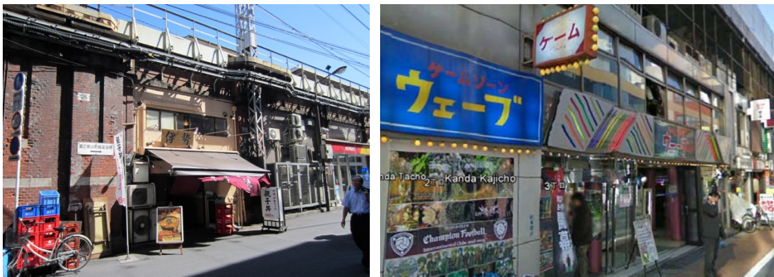
Figure 151 - Knada's viaducts west (left image) and east (right image)
