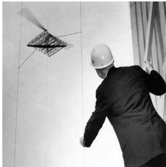
Figure 1.2 Experiment of MWPT to a helicopter
