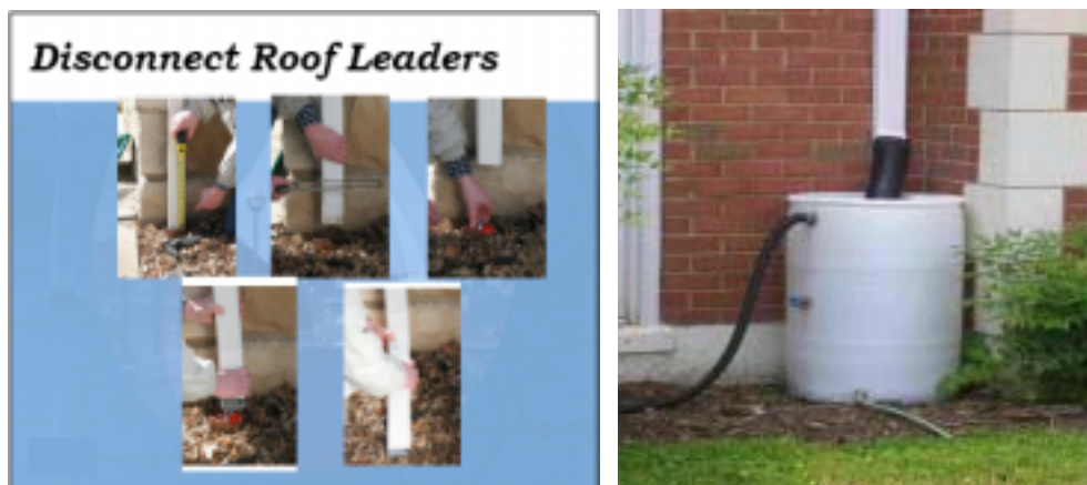
Fig.2.5. Roof leader disconnection to reduce flow to the system (Fordiani, 2006)
