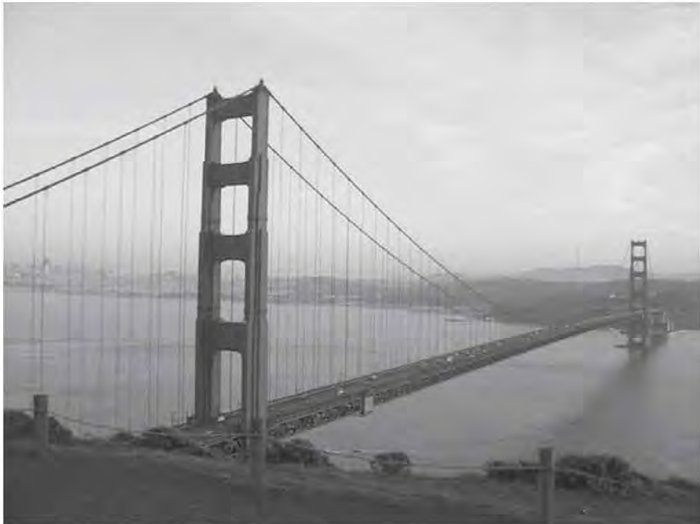
Figure 8. Golden Gate Bridge, San Francisco USA.
