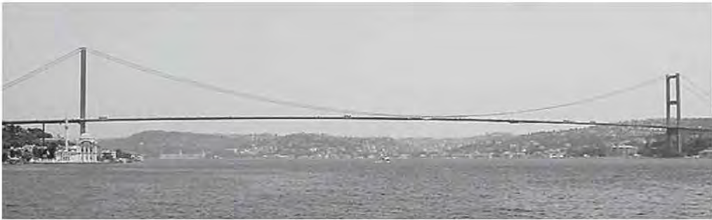
Figure 1. Bosphorus Bridge, Istanbul Turkey.
