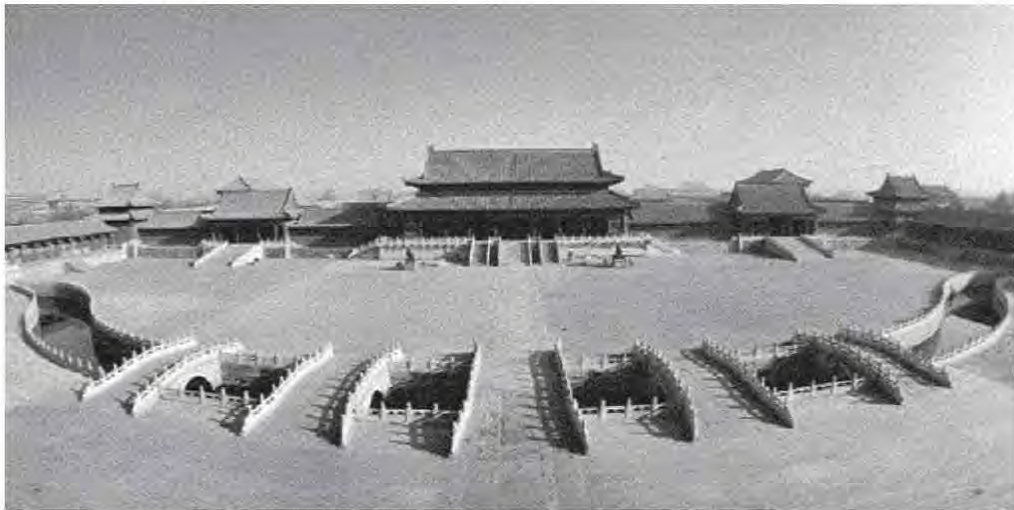
Figure 4. The Five Bridges of Forbidden City, Beijing China.
