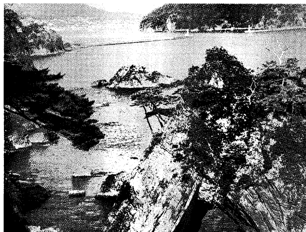
Fig. 10. Breakwater in Ofunato bay (Iwate Pref.).
