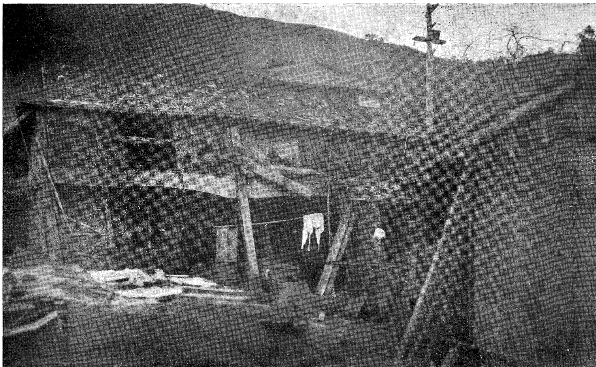
A warehouse at Kitano, Obama. Badly damaged.
