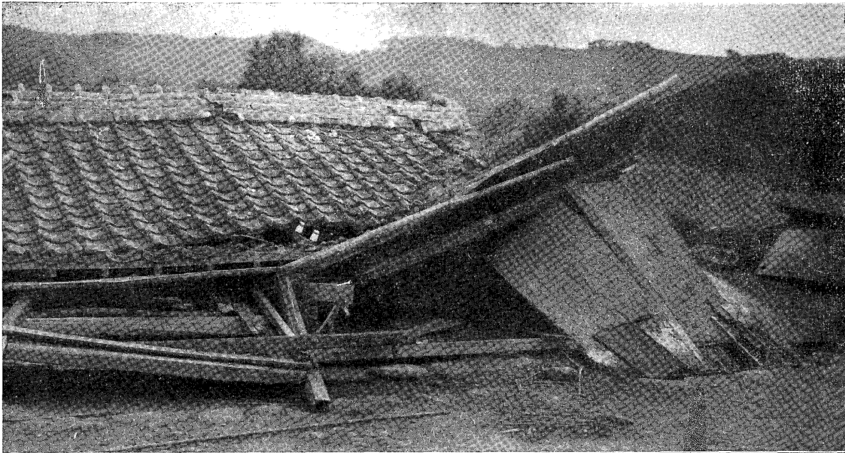
A collapsed house at Tsukanoyama, Minami-Kushiyama.
