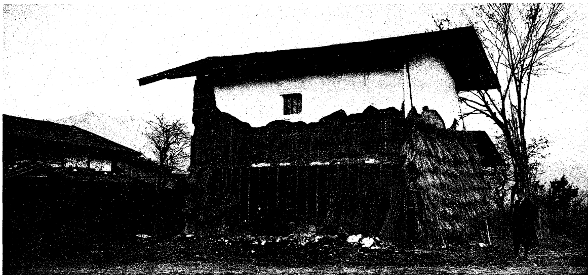
Fig. 3. A Dozo (Japanese Ware-house) at Shimizu, Tokiwa-mra, with its mud wall badly shaken down.
