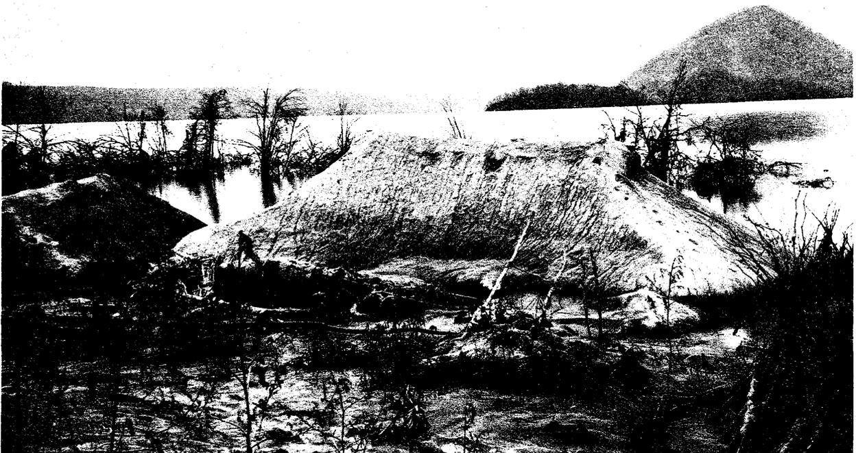
Fig. 10. A consequence of the Elevation of the new Mountain: Cottages at Pontokari overturned on account of the increasing inclination of the ground. The submerged trees show the subsidence of the shore due to the elevation of the northern slope of the New Mountain. (Nov. 10th, 1910.)
