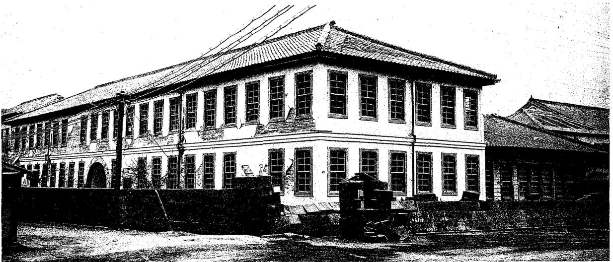
Fig. 10. Part of the Prefectural Buildings: The plasters on the E. and W. longer sides were much cracked and shaken down. The N. fence stone wall was partially overthrown.
