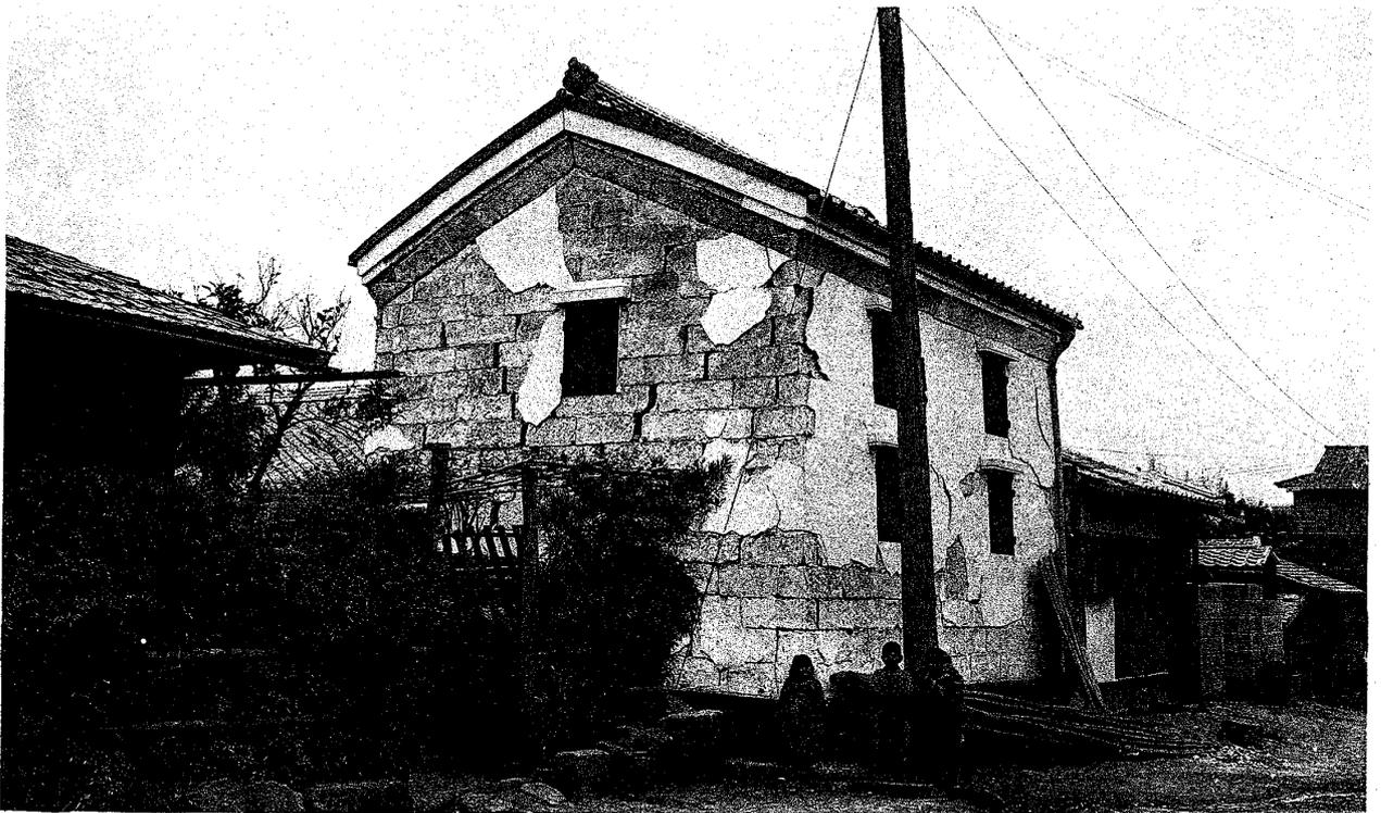
Fig. 8. A Stone Warehouse, in northern part of Kagoshima, badly cracked along mortar joints.
