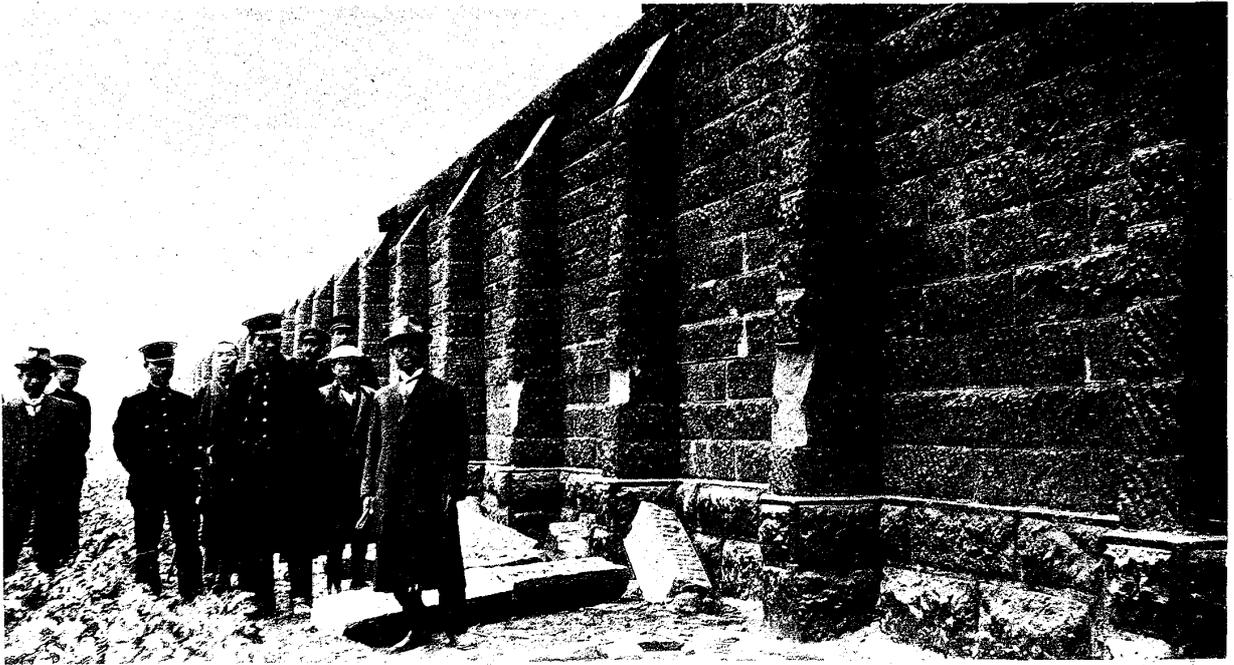
Fig. 9. Stone Fence Wall of the Kagoshima Prison. Stones below the horizontal crack line scratched off.
