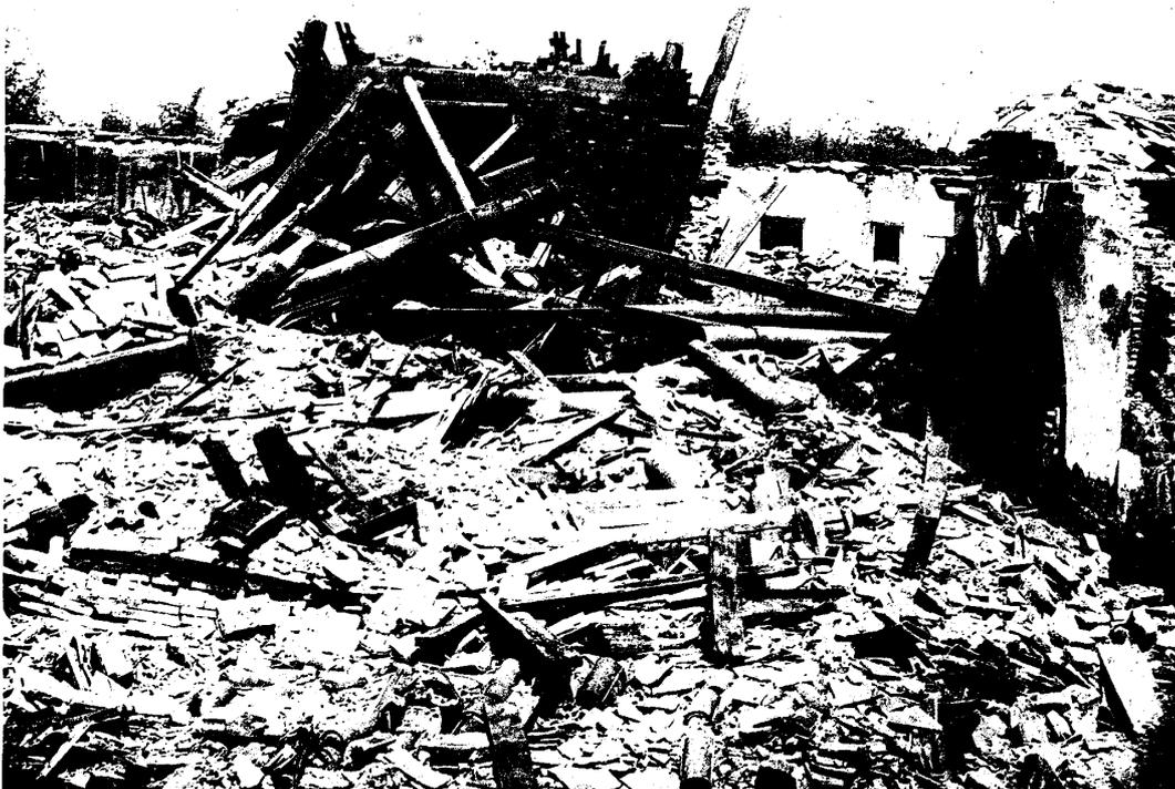
Fig. 9. The native Maso Temple, in the city of Shinko. The building was completely destroyed owing to bad masonry and weakness of wooden timbers on account of ravages of white ants.
