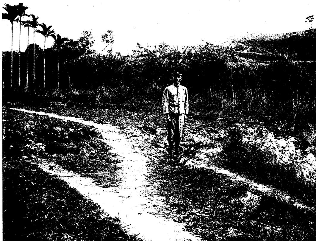
Fig. 4. Shear of the Taihorin-Baishikō Road; the foreground (southern side) sunk 6 feet and was displaced 6 feet westwards. (×) Mark the former continuation of the road.
