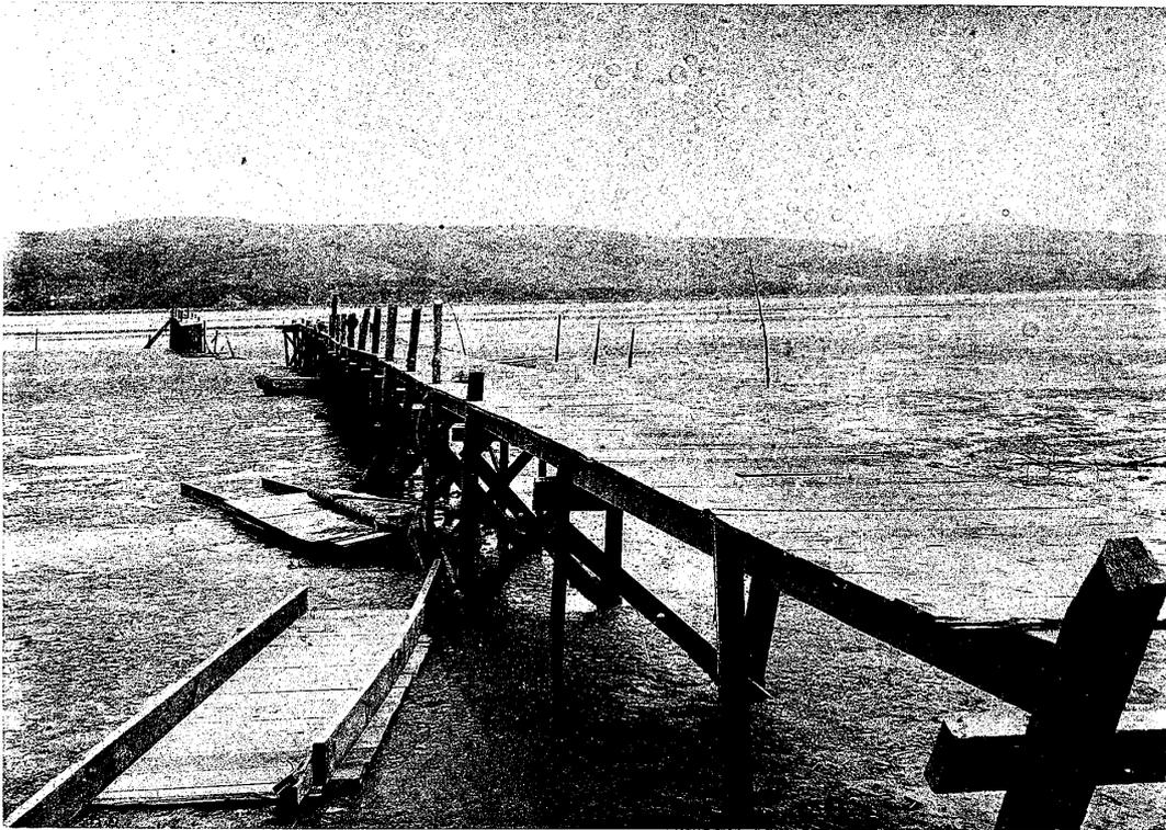
Fig. 11. The shearing effects on a pier at Inverness, on the west coast of the Tomales Bay. The end part of the pier was displaced about 20 feet towards NNW.
