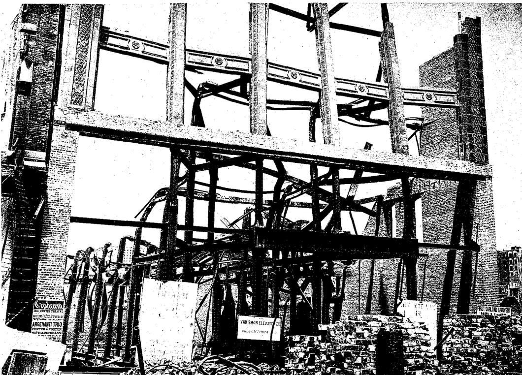
Fig. 16. The ruined condition of a steel-framed brick house in San Francisco, which was dynamited and then burnt, showing the remarkable effects of the intense heat.
