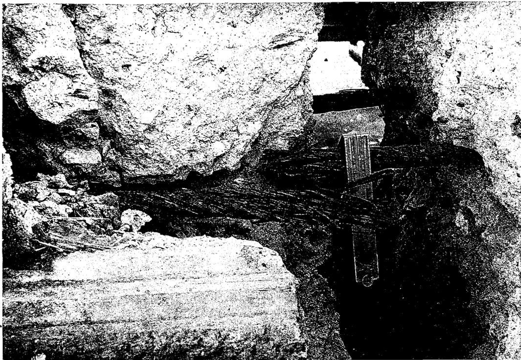
Fig. 18. One of the cracks of the basement wall. The steel cable, one inch in diameter, which was embedded in the concrete, was broken.
