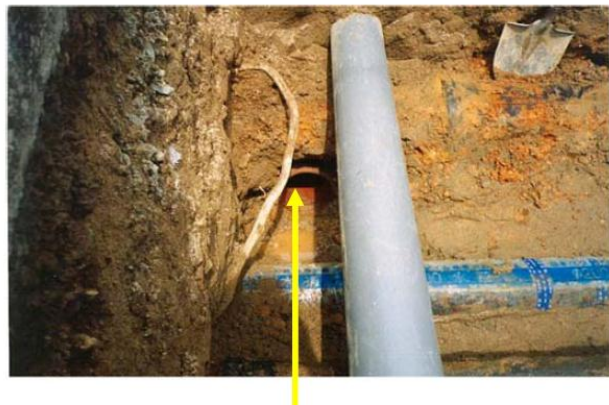
Figure 2. 14: Abundant pipe has not been properly closed or removed (Kuwano, R 2011)
