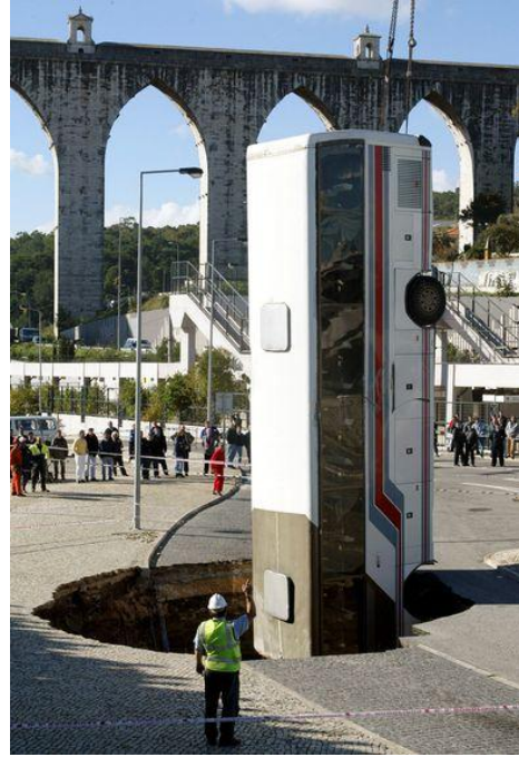
(c) Lisbon, Portugal in 2003 Cause: Damage of a sewer pipe
