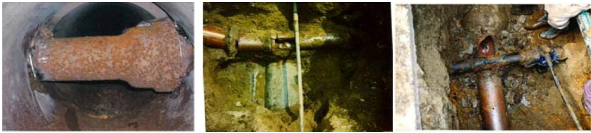
Figure 2. 12: Sewer pipes have destroyed by other pipe lines (Kuwano, R 2011)
