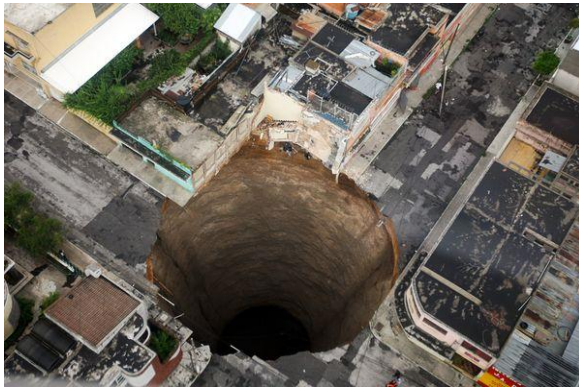
(b) Guatemala in June 2010 Cause: Heavy rain and damage of sewer line
