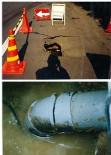
Figure 2.10: Cave-in caused by gap existed in a vinyl Chloride pipe (Kuwano, R 2011)
