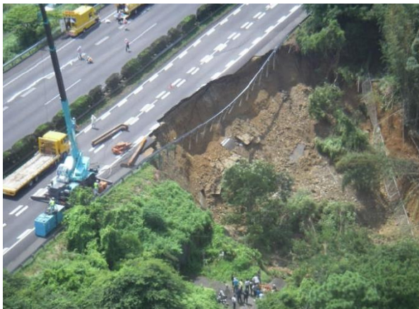
Fig.1.7. Collapsed highway embankment along Tomei expressway, Japan (Takagi et al., 2010)
