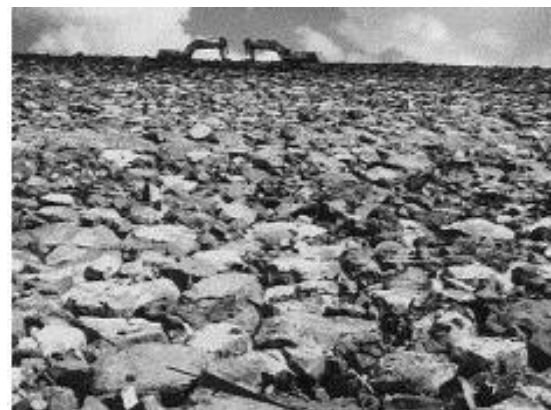
Fig.1.6. Weathered vesicular basalt blocks used in the rock-fill section of dam (Cetin et al., 2000)
