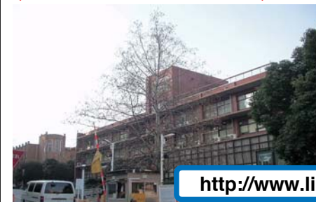
External view of the library (before reinforcement works)
