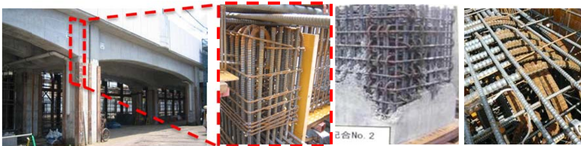
Fig. 1.1 Reinforcement congestion at beam column joint
