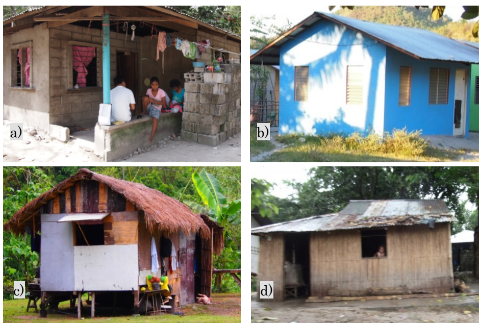
Picture 6-7. Two most frequent type of house in Target, (a) one-storey concrete house built by the owner; (b) one-storey concrete house built by GK foundation GK; (c) traditional house with modified walls (wooden boards); (d) traditional house with modified roof (met
