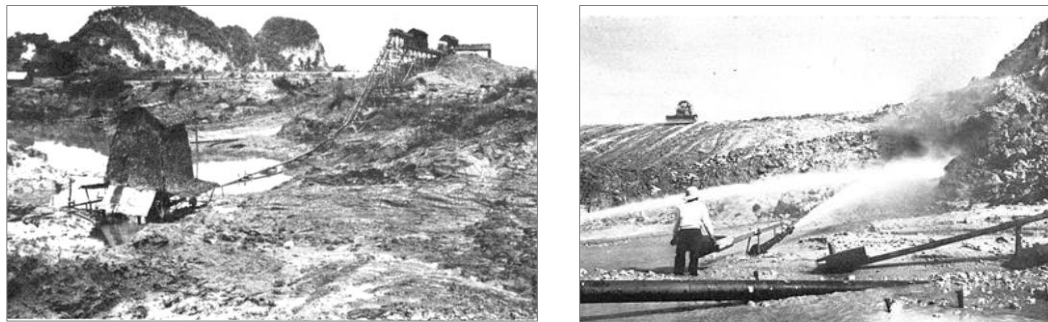
Figure 3.6: Gravel pump mining technique operated with pipelines and pump house at one of the mining site near to Ipoh in Kinta Valley district (Source: Yip, 1969).
