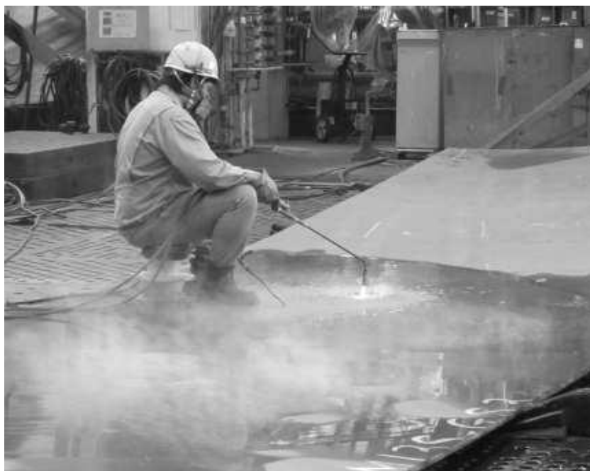
Figure 1-5 Heating forming with gas burner and water hose
