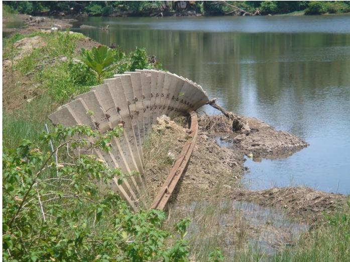
Figure 18: Heavily damaged railway embankment in due to the 2004 Indian Ocean Tsunami
