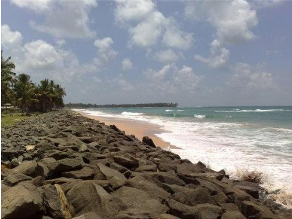
This is a beach revetment which prevents the net coast line erosion from strong wave conditions.
