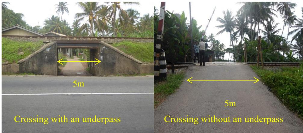
Figure 73: Railway embankment with and without an underpass
