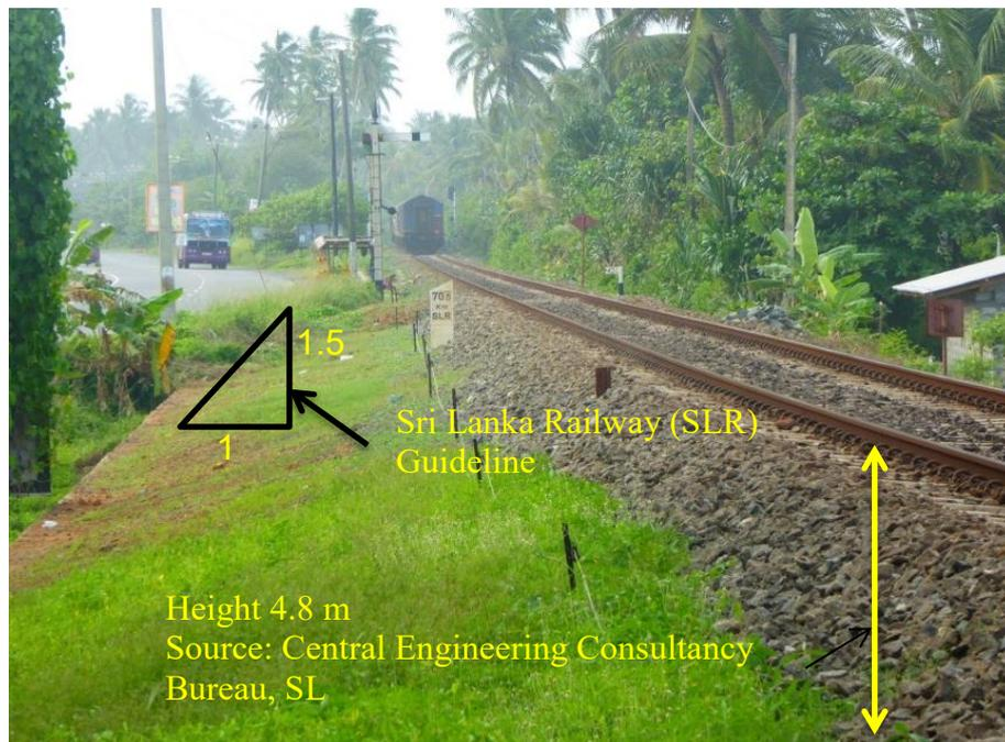
Figure 71: Picture of existing railway embankment in the case study area
