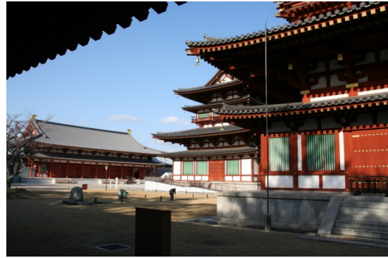
Photo 46: Yakushiji Temple, after restoration work
