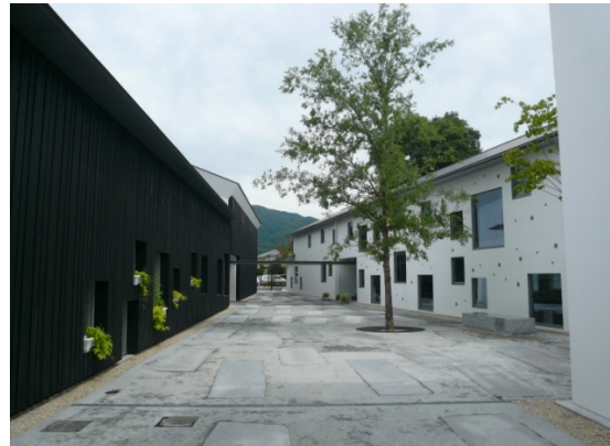
Photo 144: Courtyard (from entrance)
