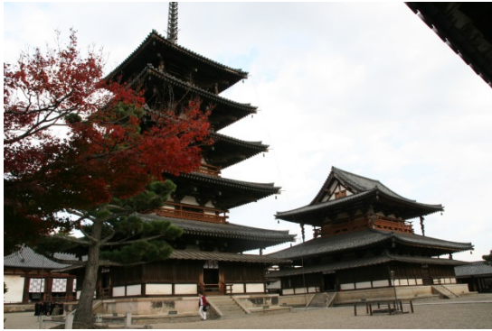
Photo 45: Horyuji Temple, the oldest wooden structure in the world from 7 th century
