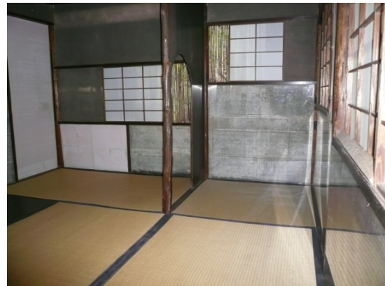
Photo 62: Placement of windows, the first priorities of which are lighting and vista effect
