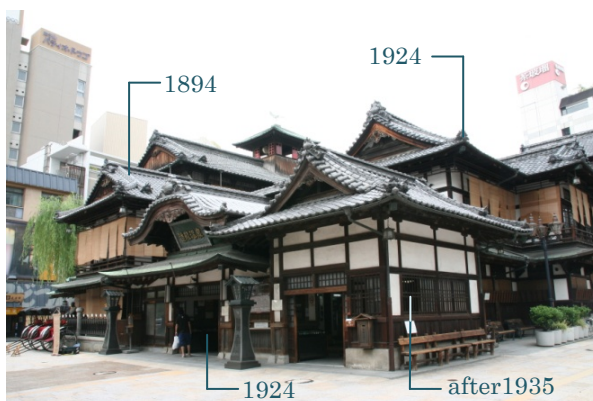
Photo 116: Main façade of the building complex
