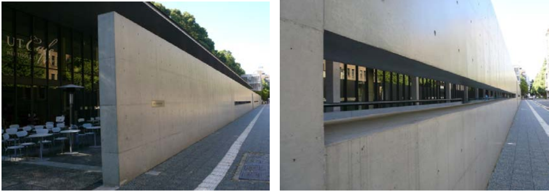
Photos 17, 18: The beauty of this fair-faced concrete finishing and the long slit on the wall show an extremely high technical level of treating concrete. (completed: 2008, location: Tokyo, architect: Tadao Ando)
