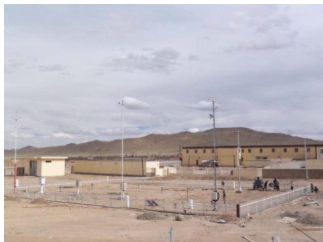
Figure 4.17 Ground status of the Gaize station in Tibet, China [玉川勝徳 et al. , 2009].
