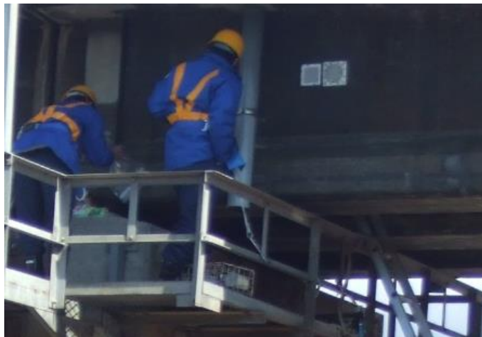
Figure 4-97 Mortar and dry gauze attached to the bridge.
