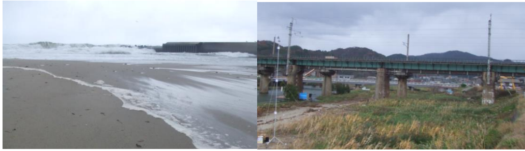
Figure 3-34 Environmental condition near exposure site.
