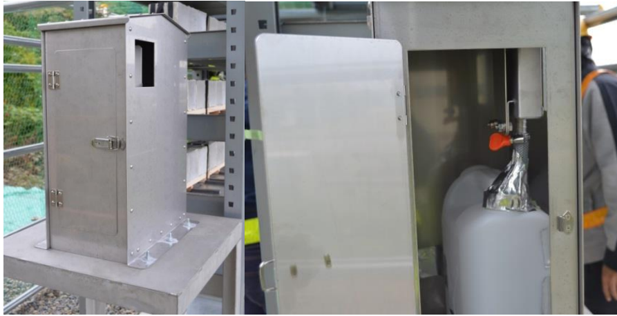
Figure 2-9 Airborne chloride capture tank and plastic container inside [19].
