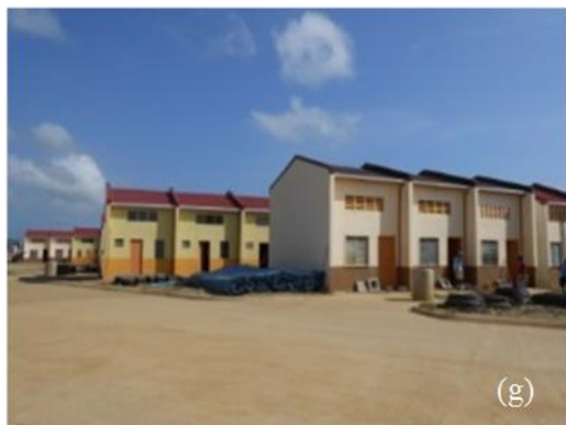
Figure 10. Photographs of Shelter Options by the Authors (a) Tents immediately after disaster (photo taken last December 2013), (b) Tacloban City Convention Centre served as Evacuation Center (photo taken last December 2013), (c) Government-funded (National Housing Authority) Bunkhouses (taken last September 2014), (d) Cali
