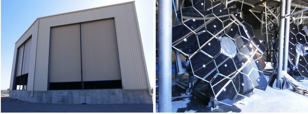
Figure 2.6: An exterior of the TA FD. (left) The overview of BR FD station. The shutters are set in three directions, which cover the FOV of four FDs each. The shutters protect the segment mirrors from sunlight, rain and dusts of the outside of the station when the observation is not performed. (right) The BR FD spherical mirror composed of 18 segment mirrors. In the figure the center position is covered for the maintenance.
