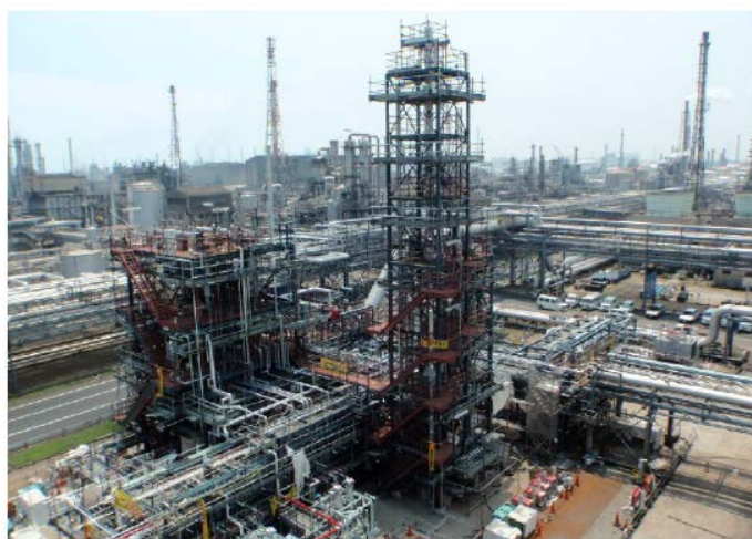
Figure 5-7 Pilot process of BTP having a capacity of 180 ton production of propylene annually
