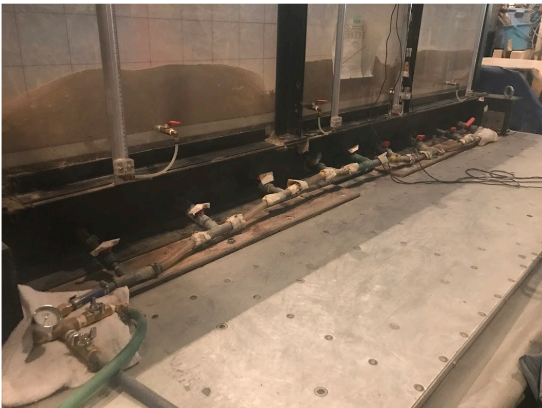
Figure 2-20. Pipes installed at bottom of soil container for water input and output
