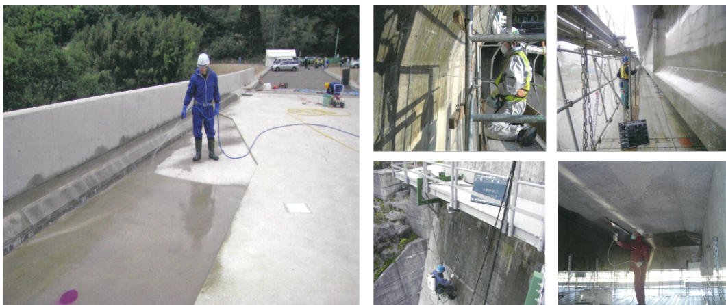
Fig2.1 Construction of Silicate-based surface penetrants
