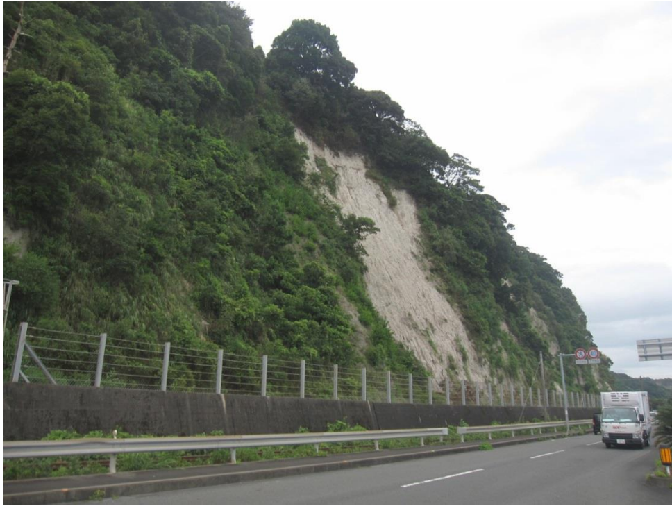
Fig. 1-1-5 Photograph of slope failure of Shirasu cliff (Photo by Ryusuke IGARASHI, August, 2012) .
