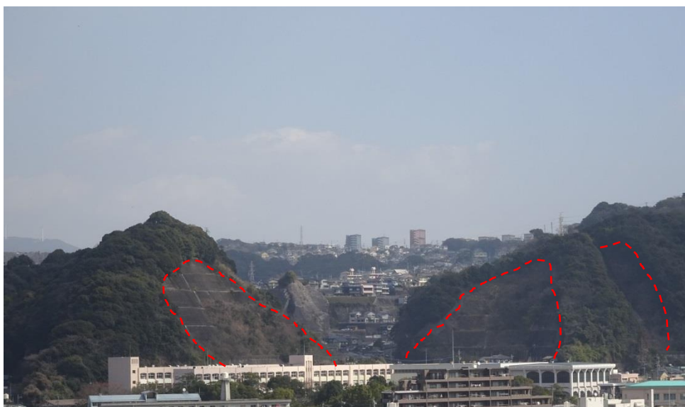
Fig. 3-1-1 Photograph showing recently failure slopes in Kagoshima city (Photo by Ryusuke IGARASHI, February, 2015) .
