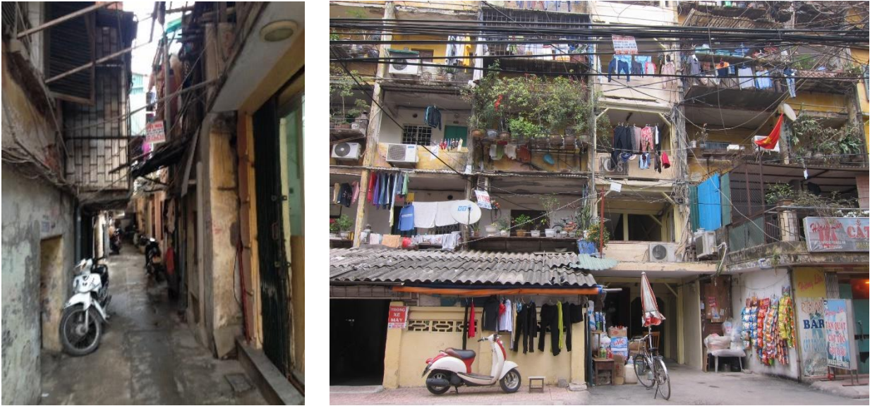
Fig. 1. 27, Fig. 1. 28: Displeasing appearance, structure failures
