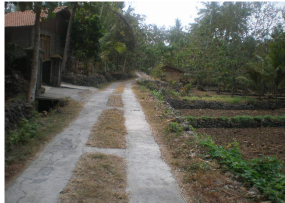
Condition of rural roads
