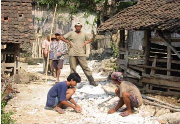
Gerakan for road repairs
