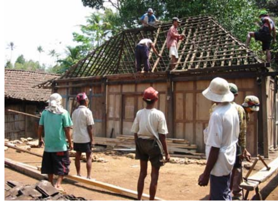
Sambatan for house repairs
