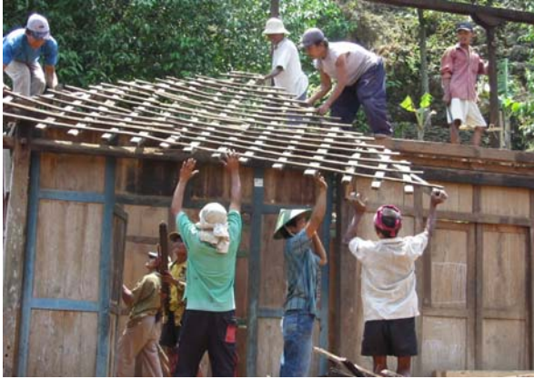
Sambatan for house repairs
