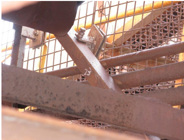
Figure 7-30 A brace attached to the walkway
