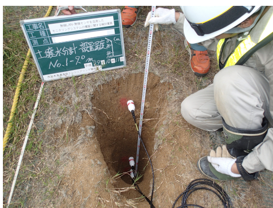
Photo 2. Installation of the soil moisture sensors.
