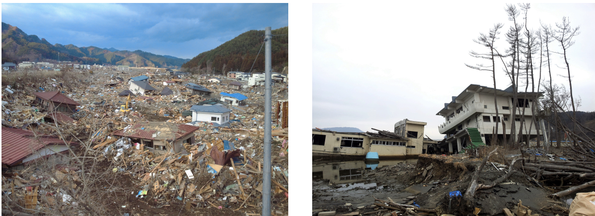
Figure 2 Damage situation (left: 1 month after in Unosumai, right: 1 year after in Nebama)
