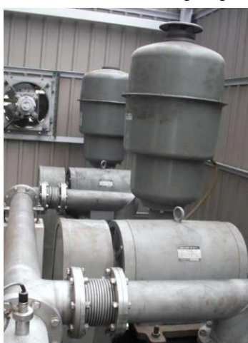
(c) Dual rotary pumps
