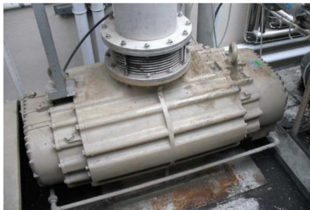
(b) A mechanical booster pump
