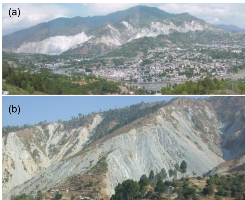
Figure 4.12 (a) Photograph showing fault rupture, slope failures and landslides behind Muzaffarabad city (b) closed up view to elaborate fault movement pattern and extent of wide brush being disturbed by the fault movement.
